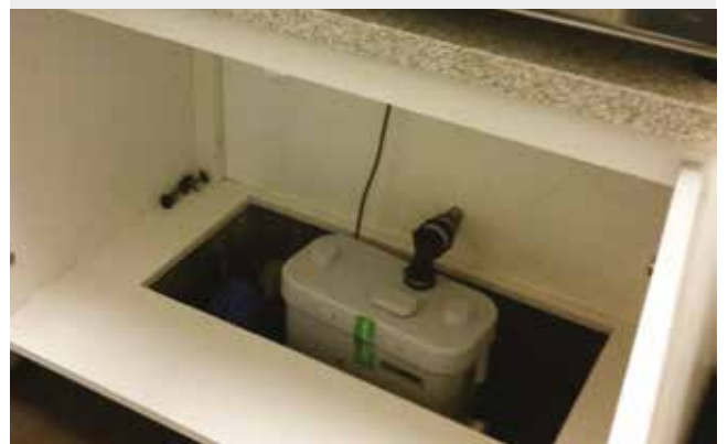
SANISPEED ® pump installed to remove kitchen waste water.
