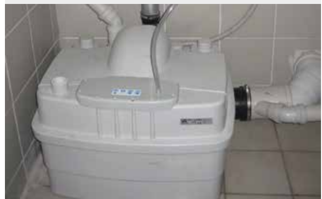
SANICUBIC® 2 Pro lifting station installed in the basement to remove waste water.
